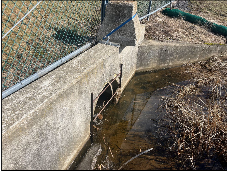
9 – Culvert inlet connecting W-1 (PEM) to drainage ditches.
