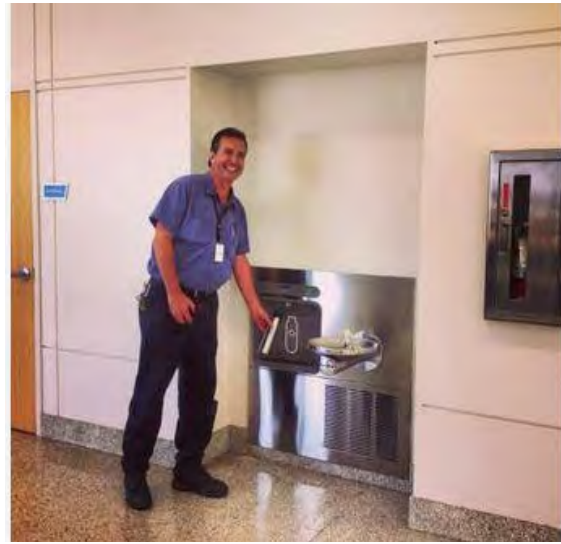
New eco-friendly water bottle refill stations installed within the terminal building
