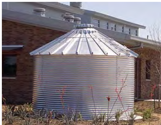
"IWS - watercache.com"; 5600 gallon commercial rainwater collection system for LEED Gold rated fire station in Denton, Texas
